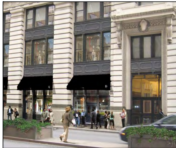
315 Park Avenue South
